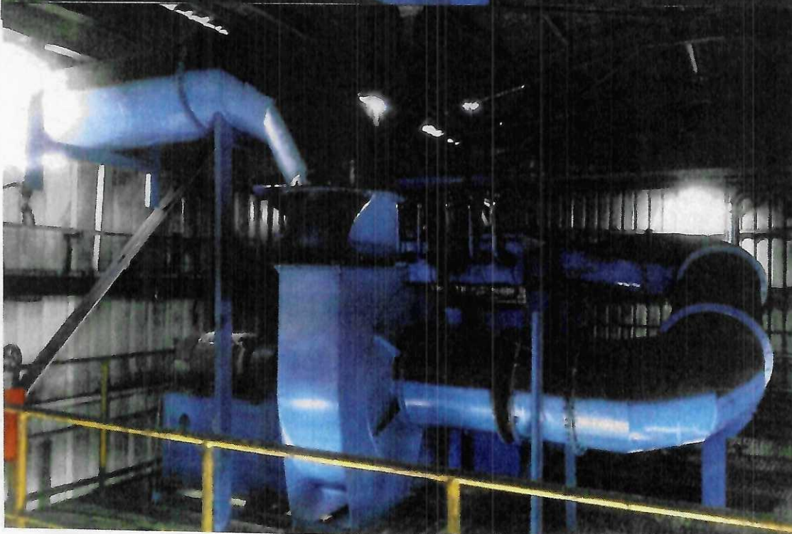
Installation of Dust - Arrester
