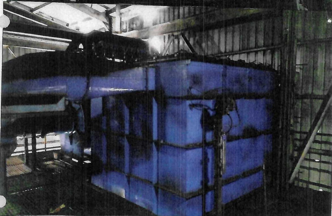
Photograph showing installation of Bag Filters of coal Crusher.
